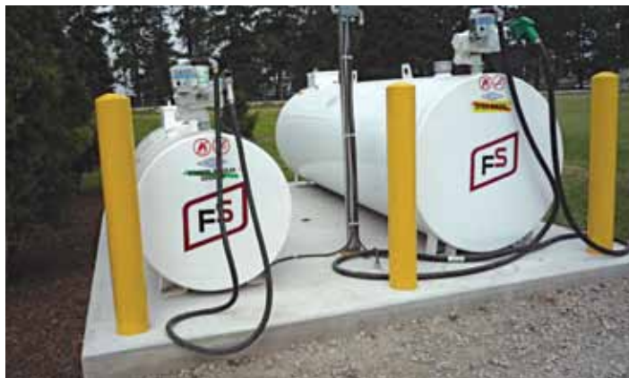
Figure 2.1. On-farm fuel storage with vehicle protection (bollards). (Photo credit: FS Partners)
