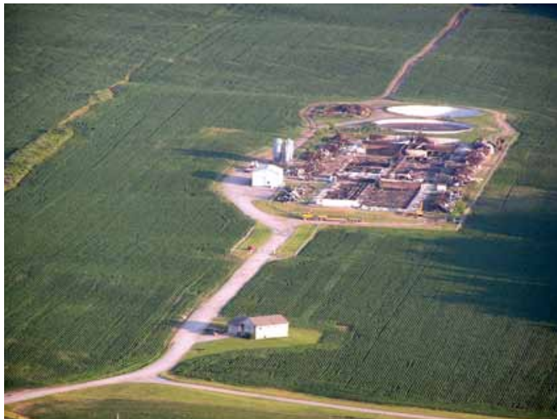
Figure 4.2. This swine facility was devastated by a fire. Note the lack of an access road completely around the buildings which hampered the ability to fight the fire.
