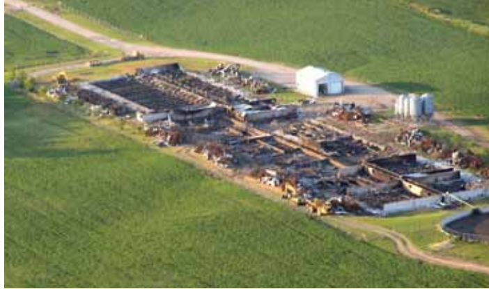
Figure 1.0. This large swine barn was completely destroyed by fire. (Photo credit: P. Stolk, Farm Mutual Reinsurance Plan)
