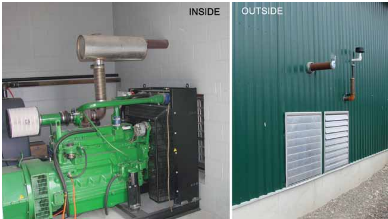
Figure 2.5. Proper installation of the exhaust pipe through the wall. Note the heat shield ring around the exhaust pipe.
