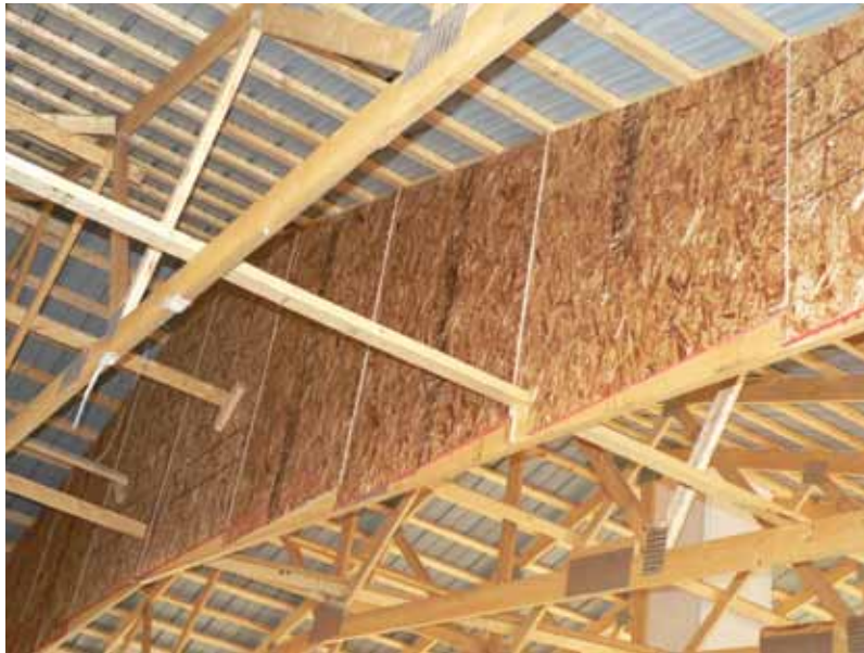
Figure 3.6. Example of an attic fire stop under construction in a new calf barn.
